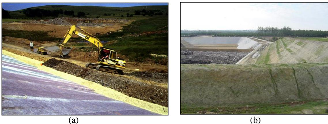
Figure 1. Example of protectives layers on GLS: (a) Selvet dam, (b) landfill.
