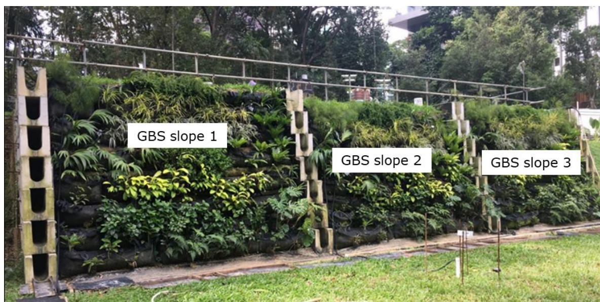
Figure 1 Pilot study of GeoBarrier System (GBS) slope in Singapore
