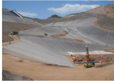
Figure 7. BGM deployment
