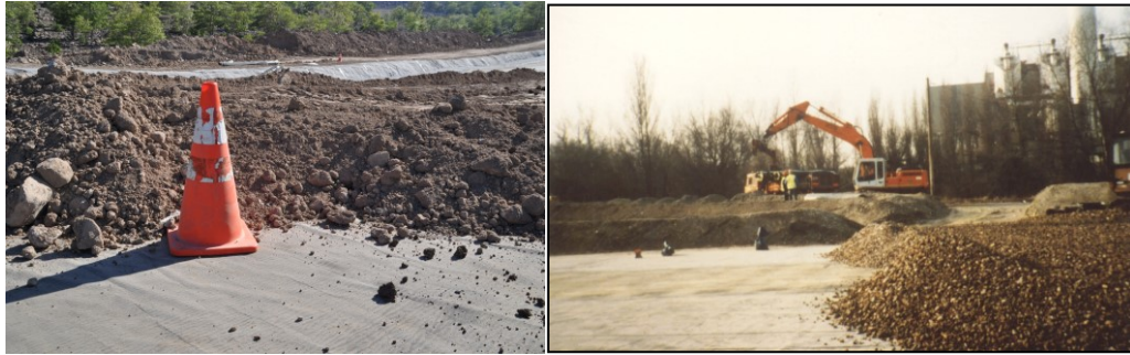
Figure 19b: Coarse grain material directly on BGM.
