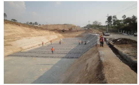
Figure 16 & 17. BGM without any wrinkle
