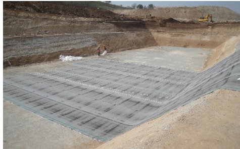
Figure 16 & 17. BGM without any wrinkle
