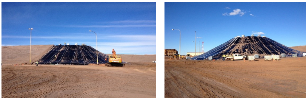
Figure 10 & 11. BGM as stockpile covers
