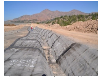
Figure 5. Leachate collector
