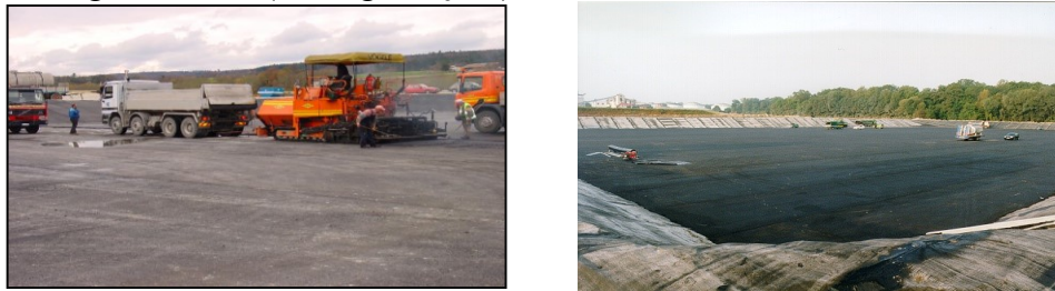
Figure 20 & 21. Asphalt concrete spread directly above BGM for cleanable tailings reservoir
