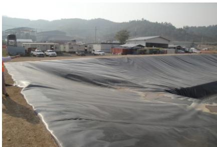
Figure 15. HDPE with wrinkles
