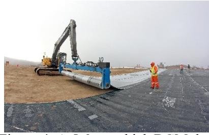
Figure 3. Large boulders removed Figure 4. A 5.6 mm thick BGM deployed
