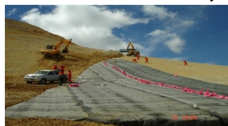
Figure 9 &10. BGM for mine waste in Chile
