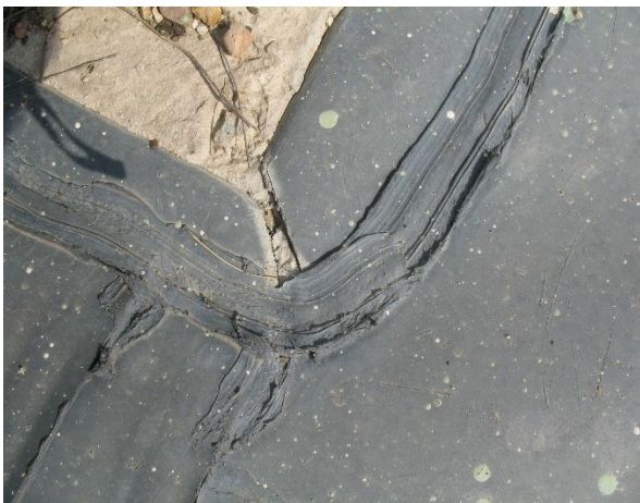
Figure 12. Joint should be welded.
