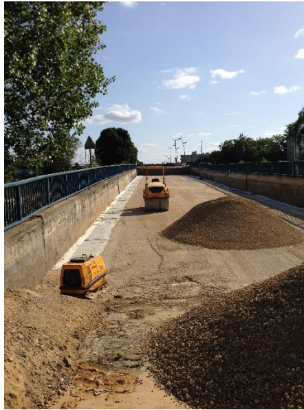
Figure 11. compacted layer before paved structure installation.
