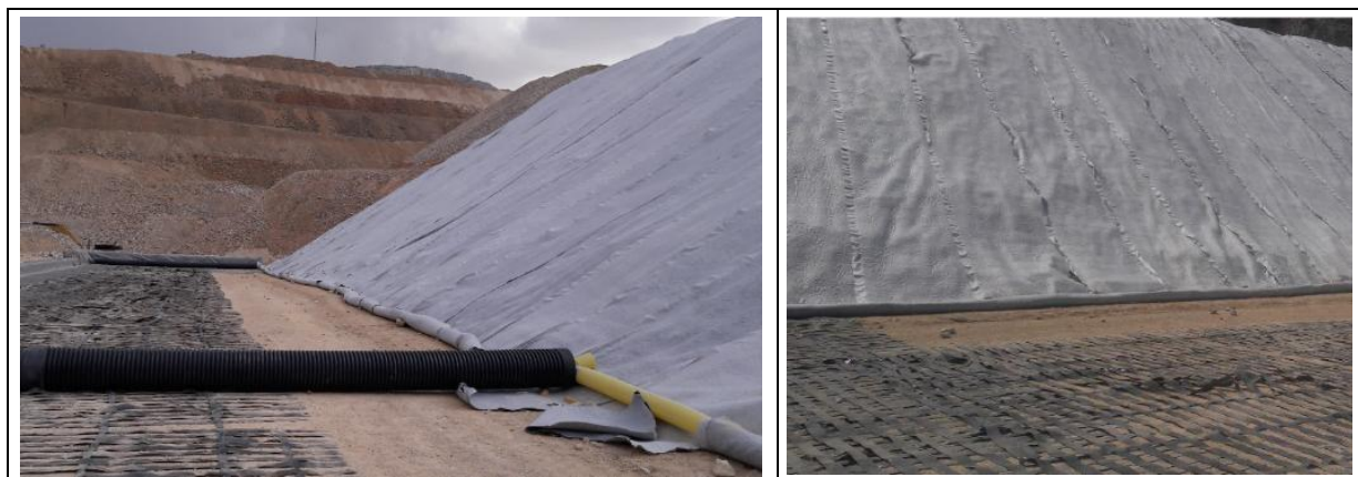
Figure 4. Drainage composite covering the slope of the crusher wall
