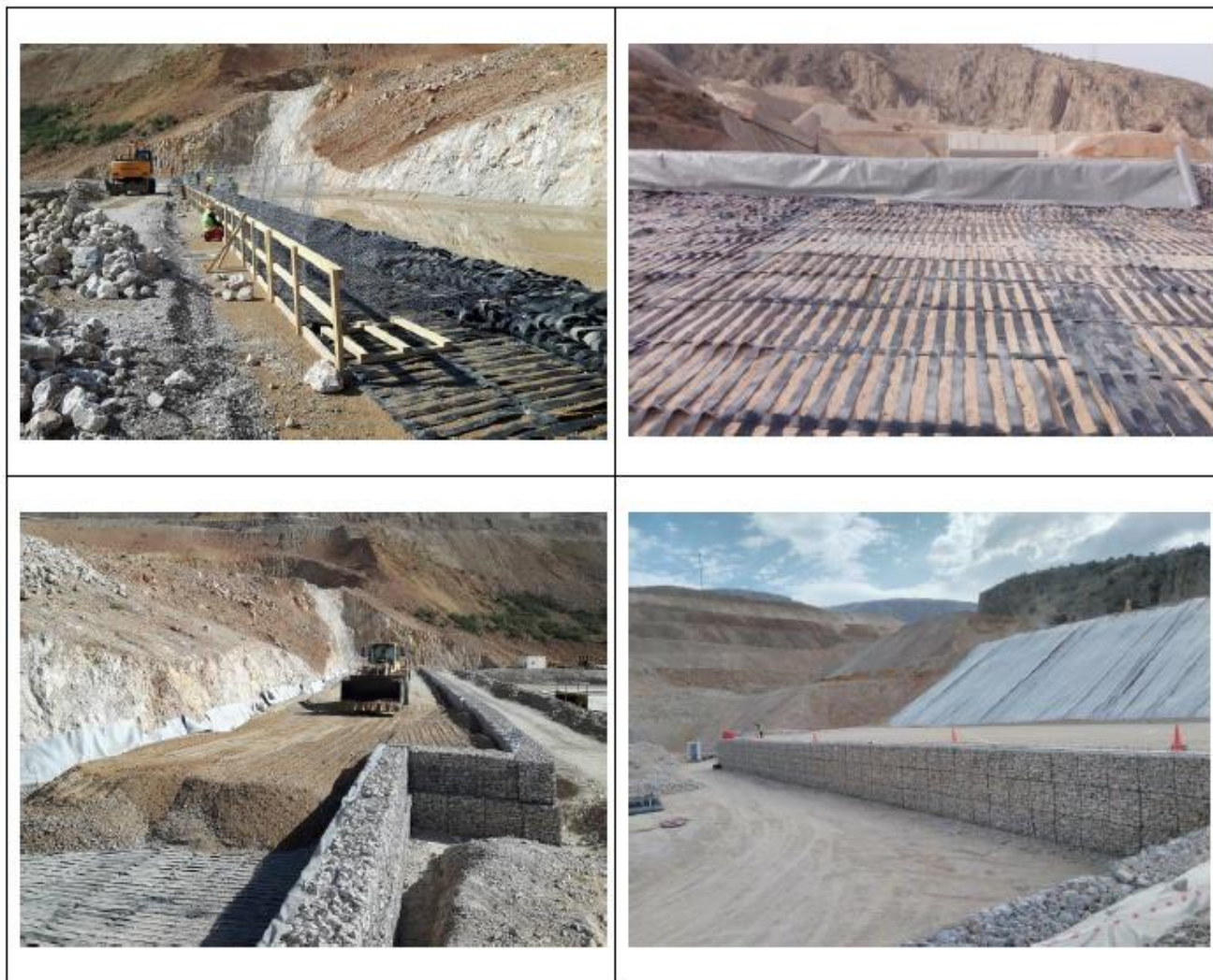
Figure 3. Various stages of the construction
