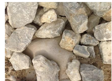
Figure 7: Suitable geotextile after first layer installation
