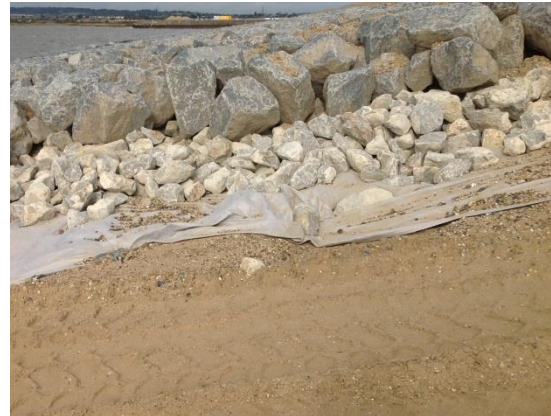
Figure 1: Rock revetment and geotextile
