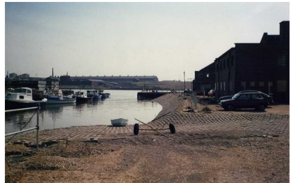
Figure 9: Flexible concrete mattress laid on filter geotextile
