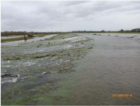
Figure 20: Flood event on overtopped embankment
