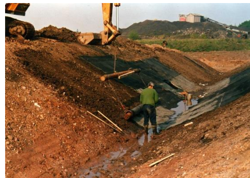
Figure 11: Open and asphalt filled TRM
