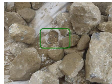
Figure 6: Site based rock drop tests & damaged geotextile
