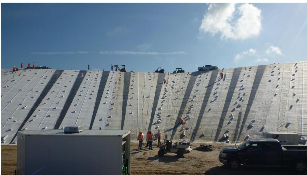
Figure 5: Placement of cover stones
