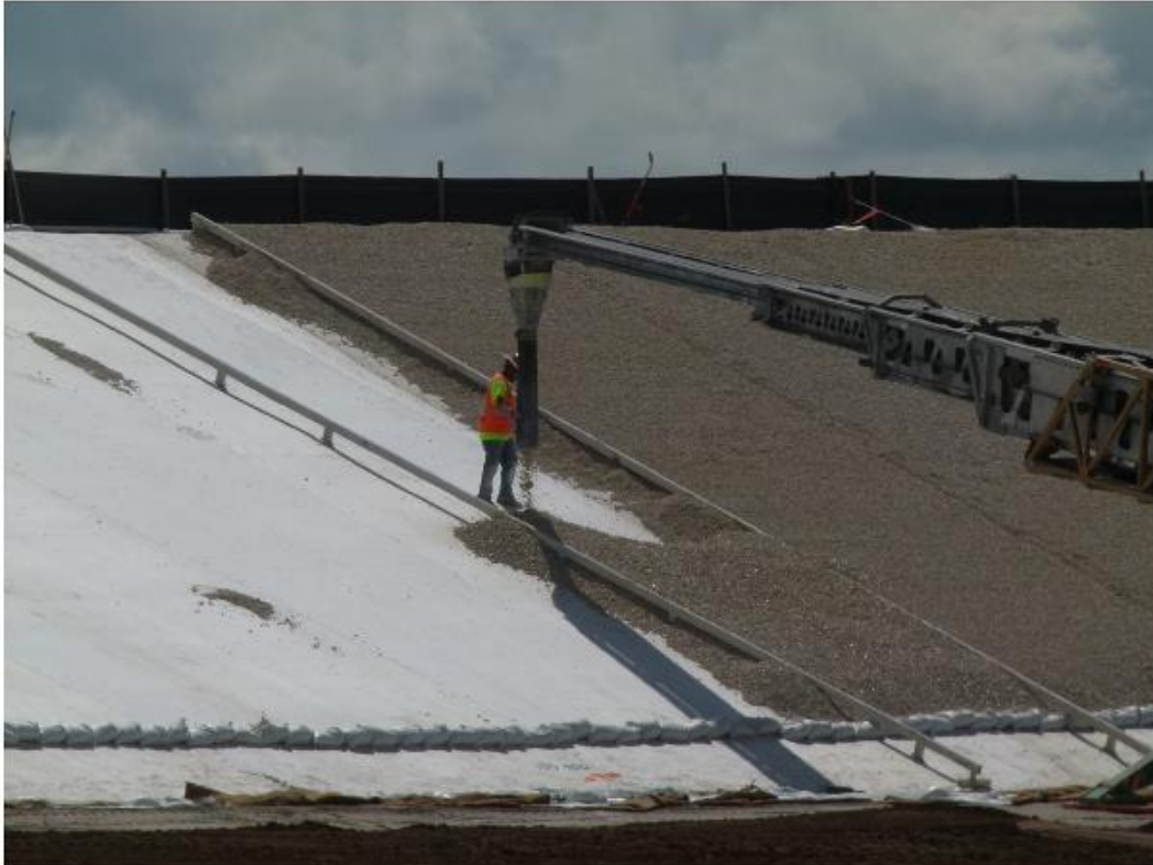
Figure 4: the laying of the geomembrane in the Bill Young Reservoir project
