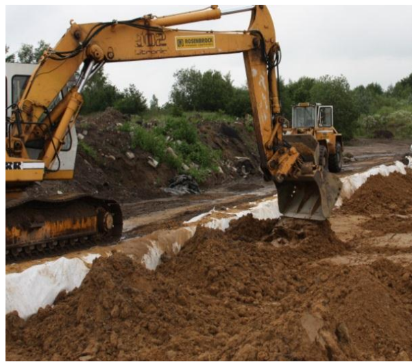
Figure 2: Side installation of the glacial till (in layers)
