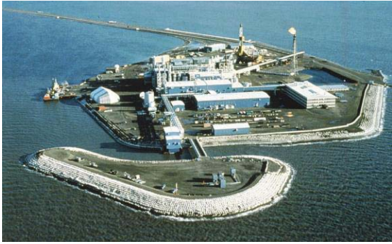
Fig. 17 Aerial view of geobag revetment protecting Endicott Island
