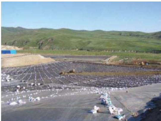
Fig. 4 Heap leach pad system lined with LLDPE geomembrane (Ng and Qi, 2012)
