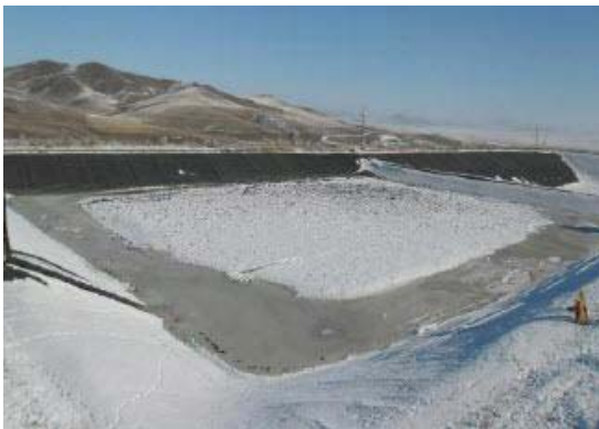
Fig. 3 HDPE geomembrane lined chemical solution pond (Ng and Qi, 2012).
