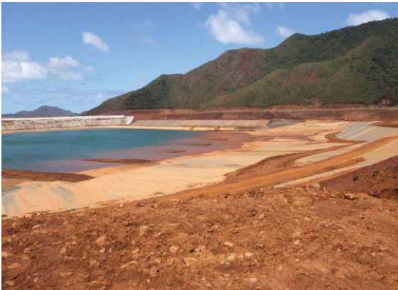
Fig. 7 A large tailings storage with various earthen structures on top of the liner. These structures can be for access or for ballasting of the liner against wind uplift and storm damage.
