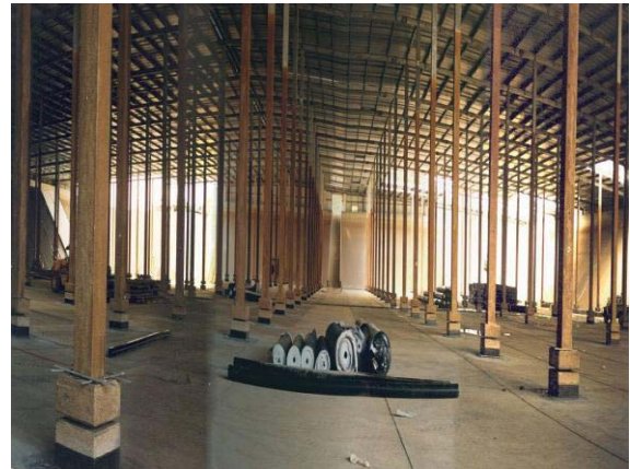
Fig. 9 Tamworth Hill reservoir with 200 columns in the floor
