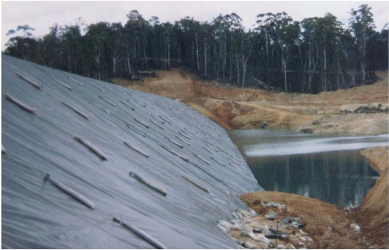
Fig. 6 A tailings dam with ballasted geomembrane on the dam face
