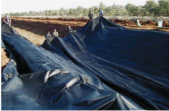
Fig. 19 Unreinforced PP 0.75 mm (Note large crew size)
