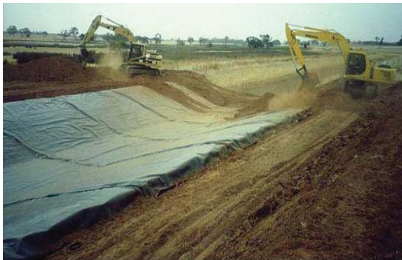
Fig. 16 Soil Cover Installation over 0.75 mm HDPE
