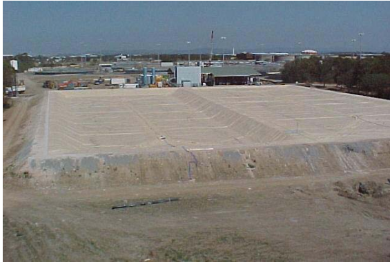
Fig. 31 Hybrid HDPE/mPE-R Covers. Note hinges same colour as main plates.
