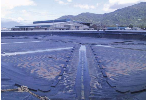
Fig. 24 An anaerobic wastewater processing facility with floating cover and gas collection
