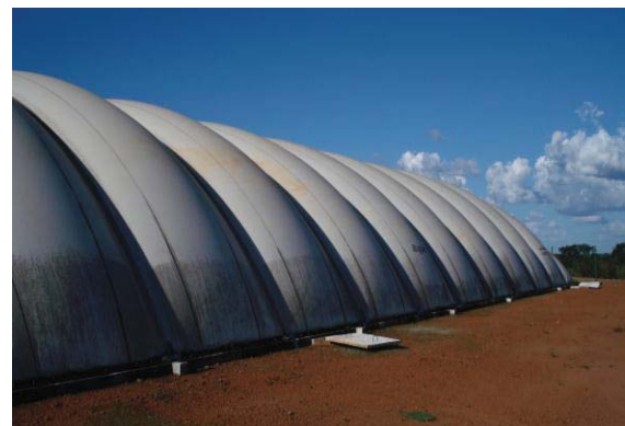
Fig. 30 An inflated gas storage cover over an anaerobic lagoon
