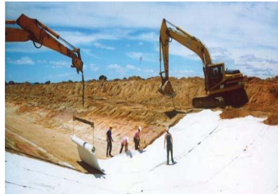
Fig. 17 GCL Installation
