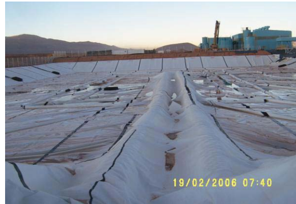
Fig. 35 Completed floating cover for a copper mine PLS pond
