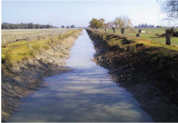
Fig. 15 Typical Unlined Channel
