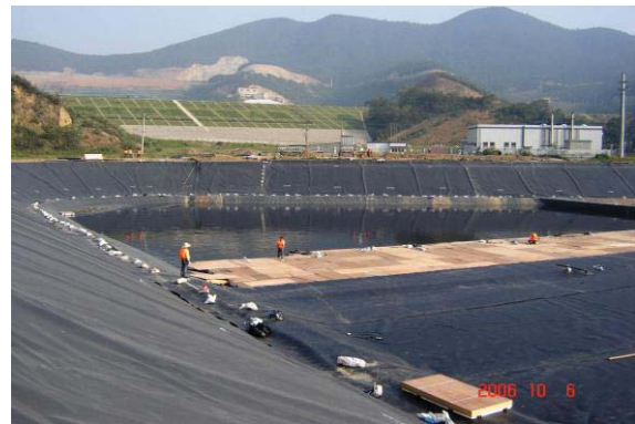
Fig. 29 A cover being built over a temporary pontoon platform.
