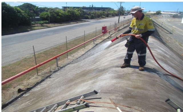
Figure 2. Application of water onto an installed GCCM – begins the curing process
