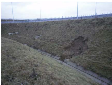
Fig.1 The cavity on the slope (junction „Piekary”) in 2013 and wireless possibility to recording events.
