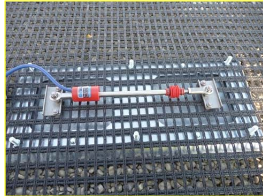
Photo 4. The view of the sensors installed on geogrid
