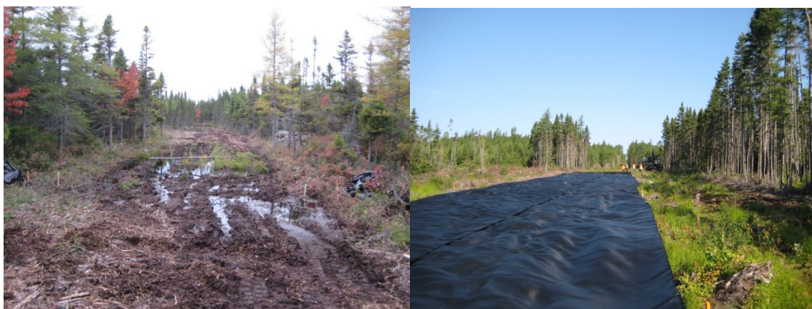
Figure 3 – fields inaccessible w/o the right geosynthetic
