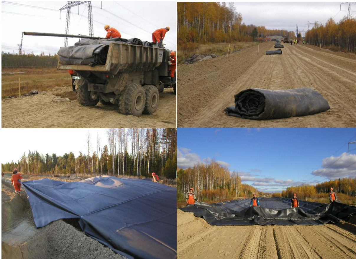
Figure 4 – prefabricated panels delivered and unfolded on site
