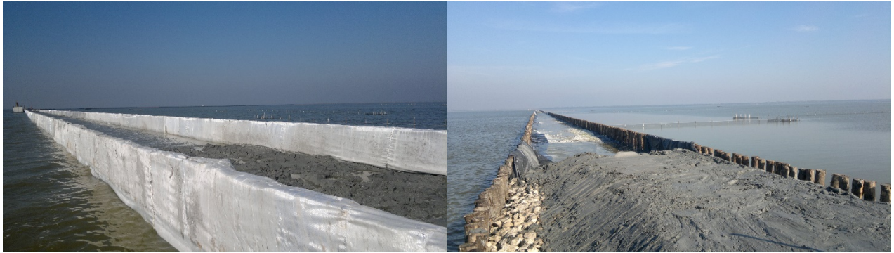
Figure 6 – unrolling and filling of the embankment
