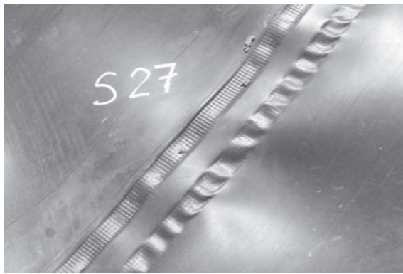
Figure 6. Example of poor nip roller tracking in a HDPE wedge weld [Scheirs]
