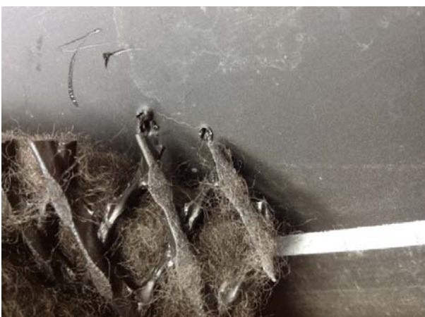
Figure 21. Sharp cut end of geonet causing puncture of geomembranes [Scheirs]
