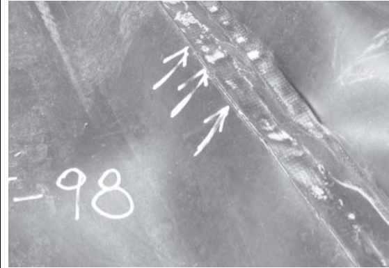
Figure 7. Example of overheating a HDPE Weld [Scheirs]
