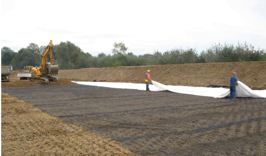
Figure 3: Second layer of reinforced soil and temporary levee in the background
