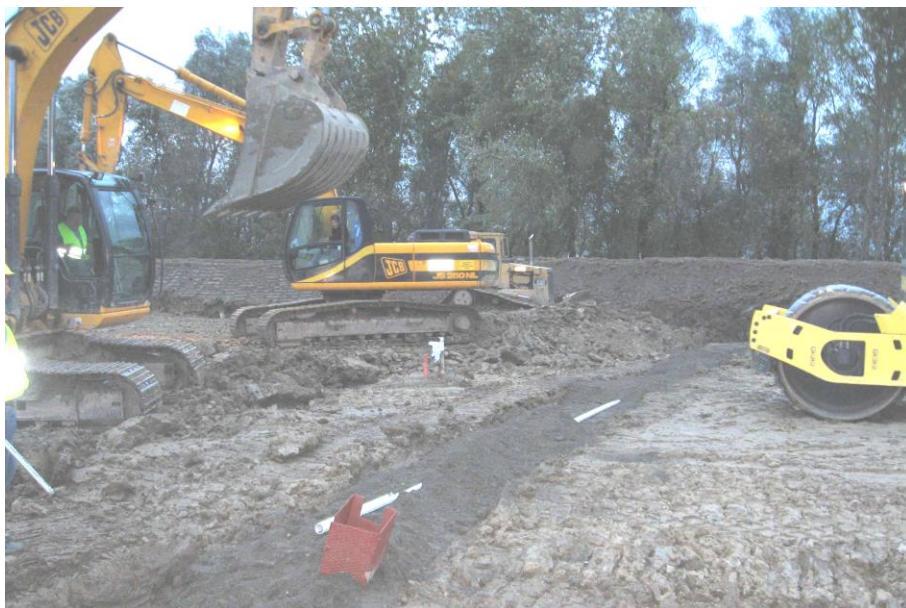
Figure 9: Installation of horizontal inclinometer
