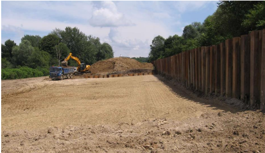
Figure 6: Sheet pile coffer dam at beginning of remediation
