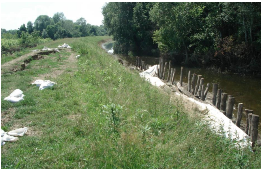
Figure 2: Levee landside slope sliding in village Račinovci
