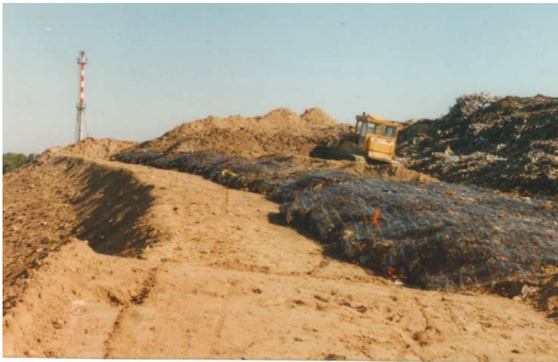
Fig. 2 The process of geogrid installation on the landfill (1993)
