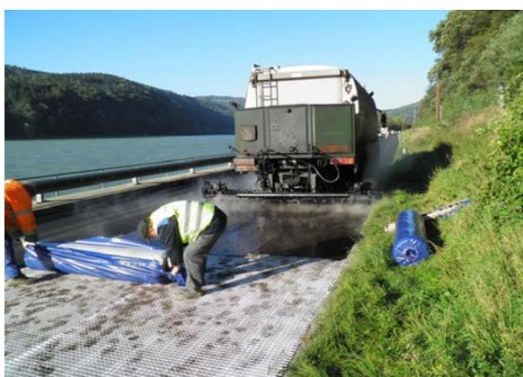
Fig 5 Spraying of tack coat
