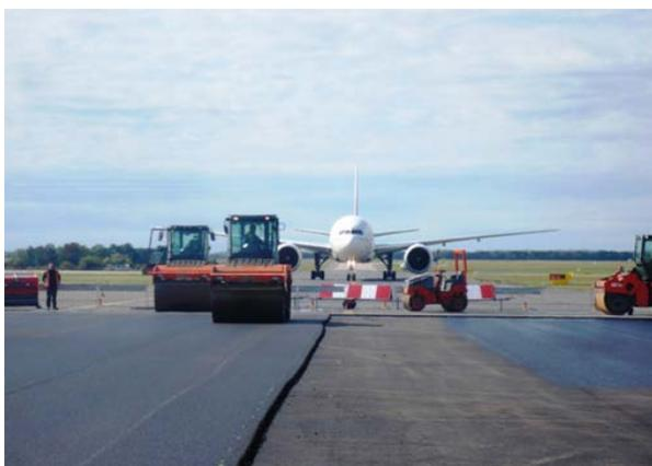
Fig 8 compaction of surface course
