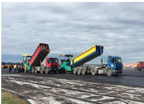
Fig 7 Installation of surface course
