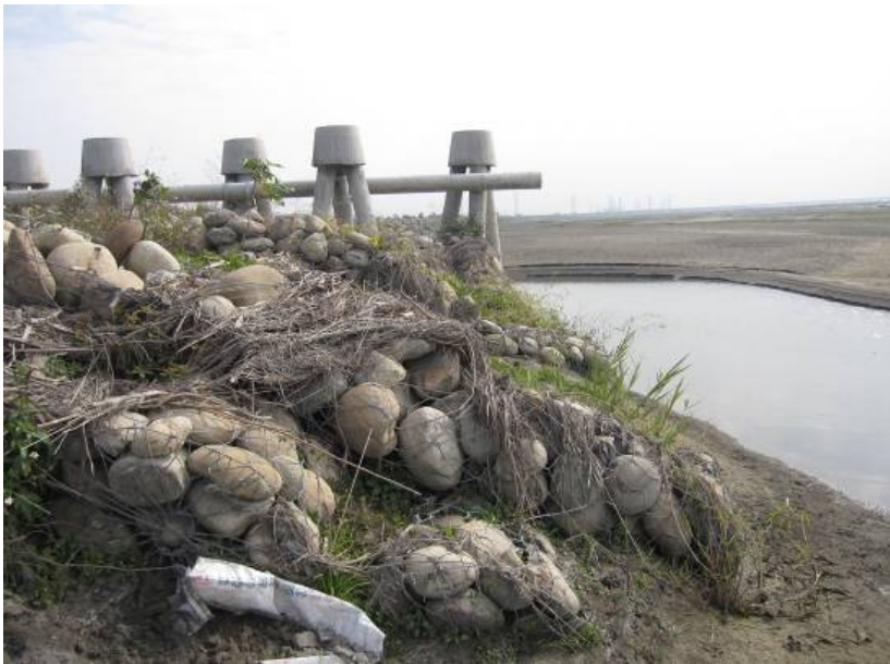
Fig. 3-3 Gabion Failure
