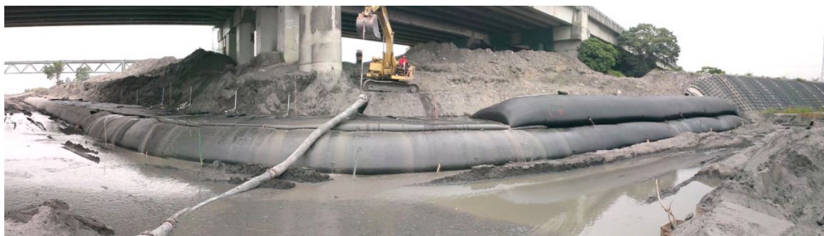
Fig. 4-2 Construction (Curve Section)
