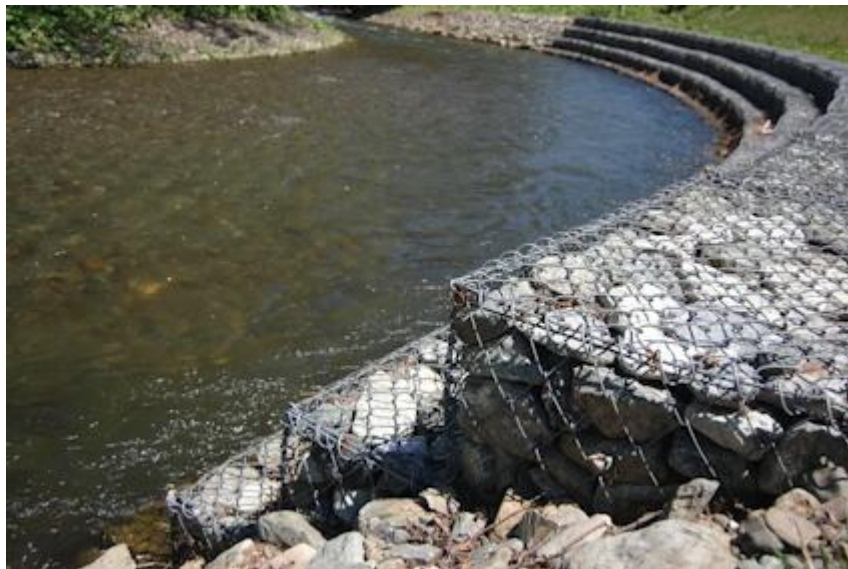
Fig. 2-3 Gabion (photo by website)
