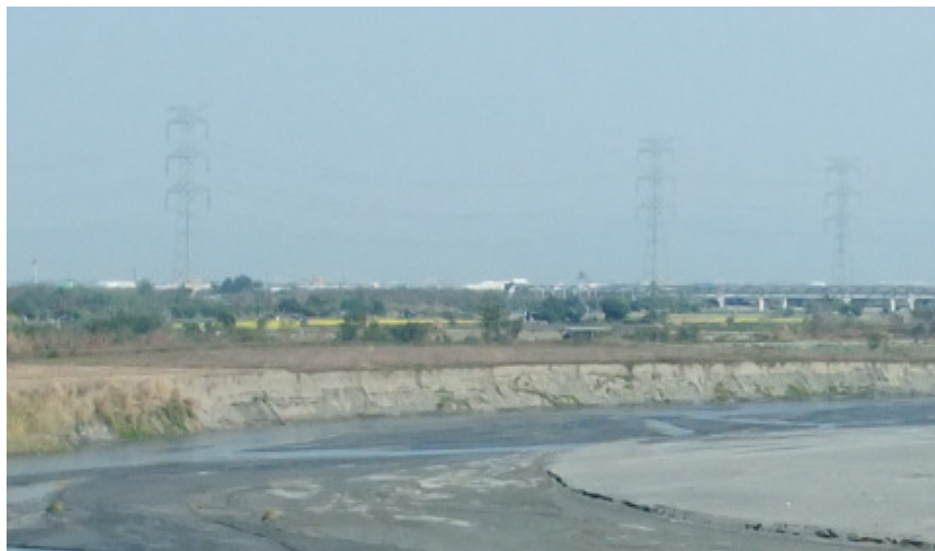
Fig. 3-2 Erosion by Flood
