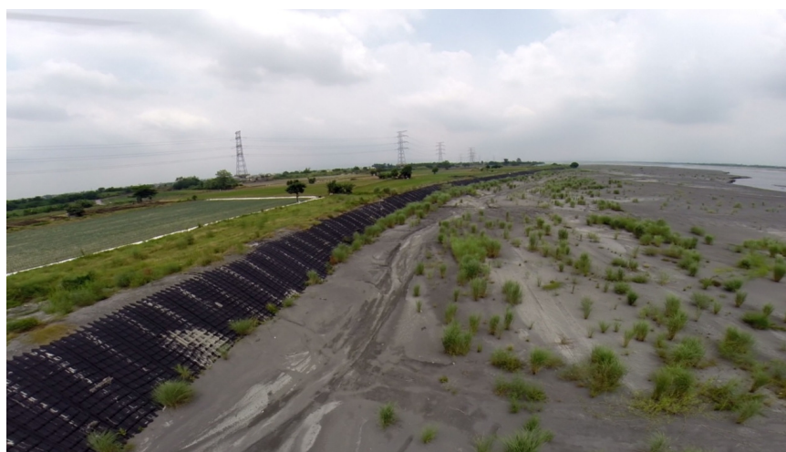
Fig. 4-4 After Construction by ACEFormer™
