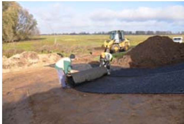
Fig. 4 Installation of beaver netting
