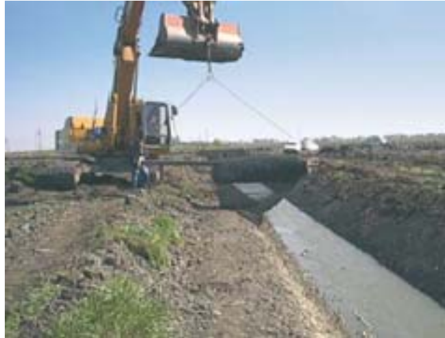
Fig. 5 Installation of beaver netting along Canale Zabarelle
