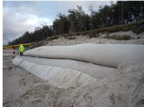
Photo 4. SoilTain® tubes after filling (photo Inora - 6.11.2012)
