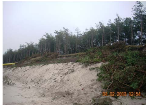
Photo 6. SoilTain® geotextile tube covered by sand brushwood and stones (photo Inora - 4.02.2013)
