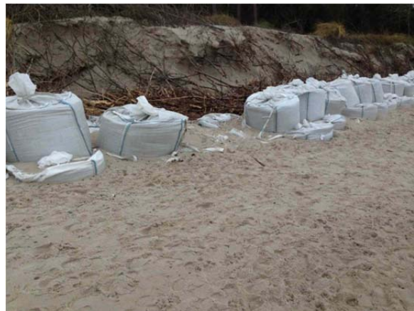
Photo 8. The destruction of sand dunes on the beach after the passage of storm Xavier - see bags filled with sand used as temporary protection (photo UM Slupsk - 27.12.2013)
