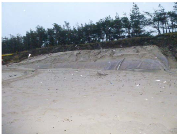
Photo 9. SoilTain® geotextile tubes after storm Xavier, 27.12.2013 (photo UM Slupsk)
