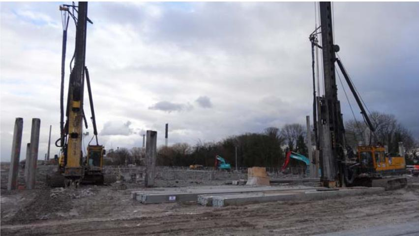
Figure 8. Piling dig rig machines on site during operation (January 2016)
