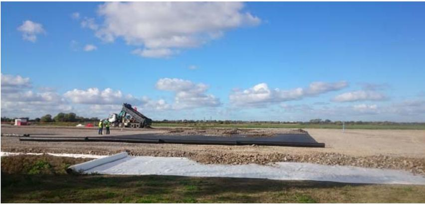
Figure 7. Multi-layer geosynthetics reinforced granular working platform during installation (October 2015)
