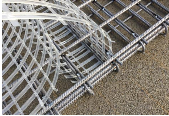
Figure 7: Implementation of the high-strength geogrid to the concrete reinforcement of the panel during the precast process
