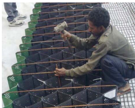
Figure 9 Laying of geogrid and geocell
