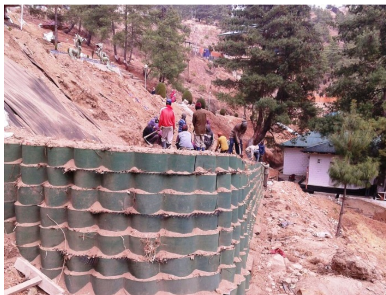
Figure 11 Green appearance of reinforced soil wall
