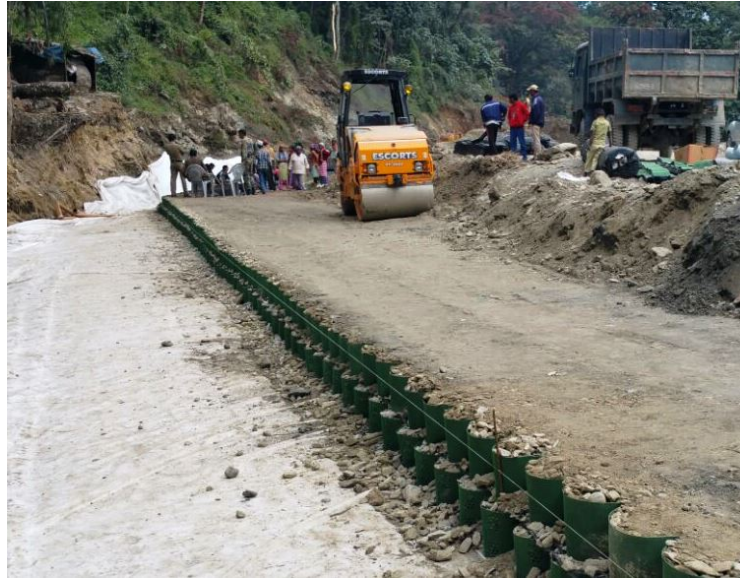
Figure 10 Infilling and compaction
