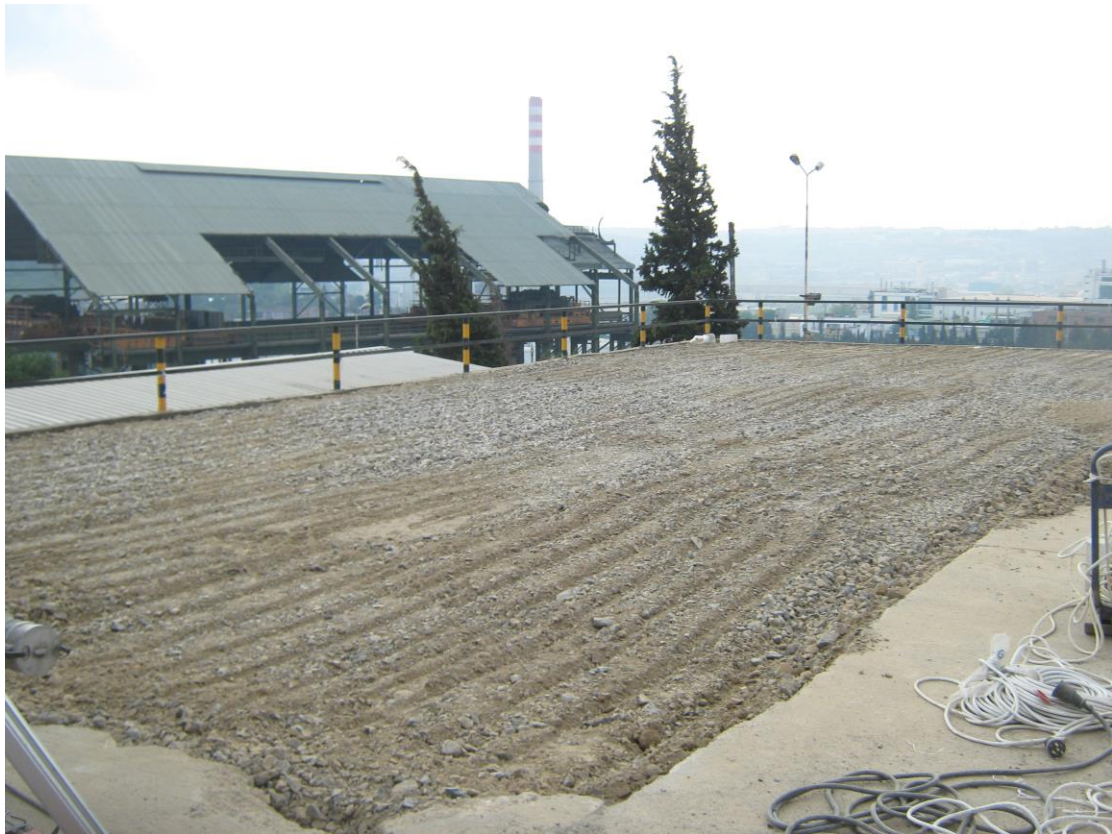
Figure 13: Placement of top layer of granular fill
