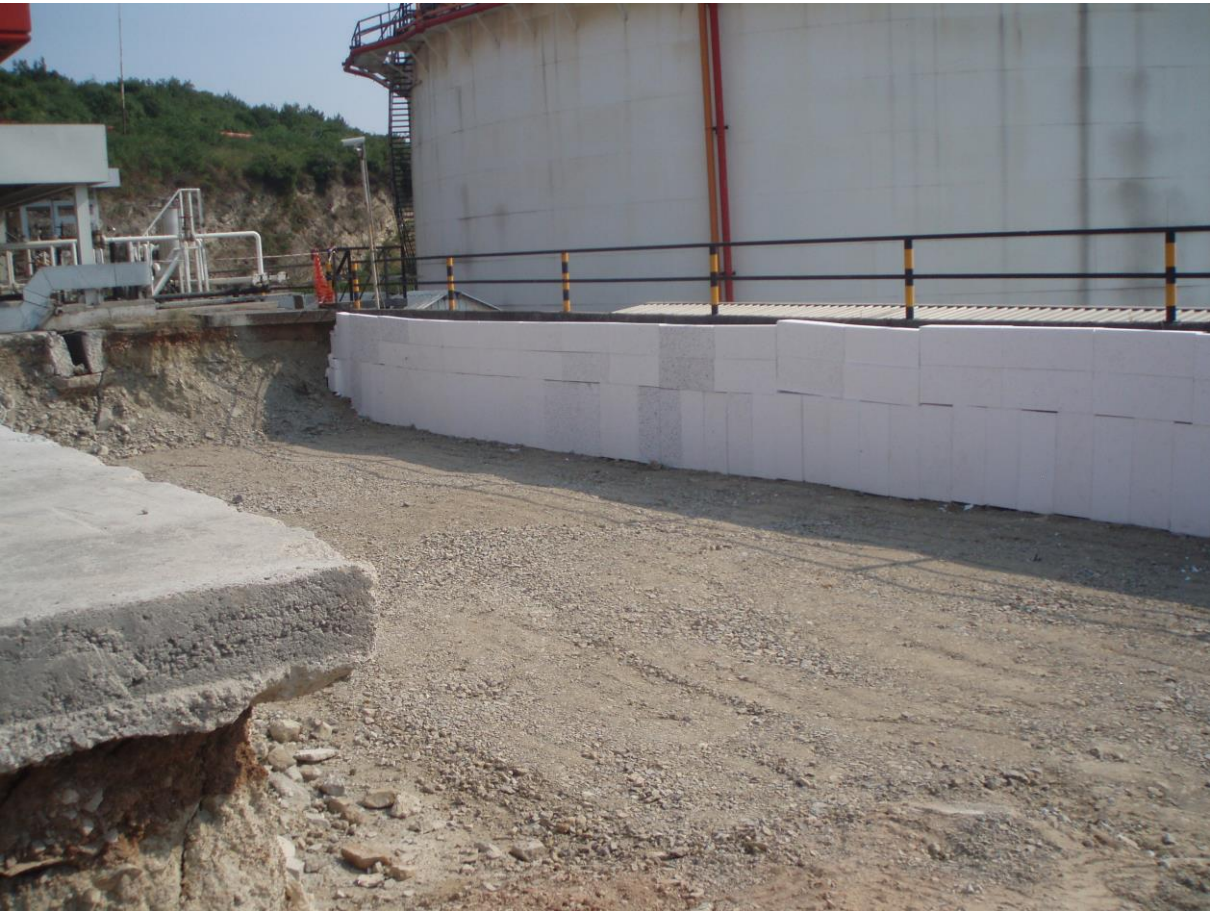
Figure 10: Placement of XPS foam boards after cleaning the site from grout
