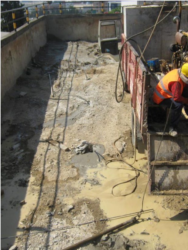
Figure 9: Grout injection
