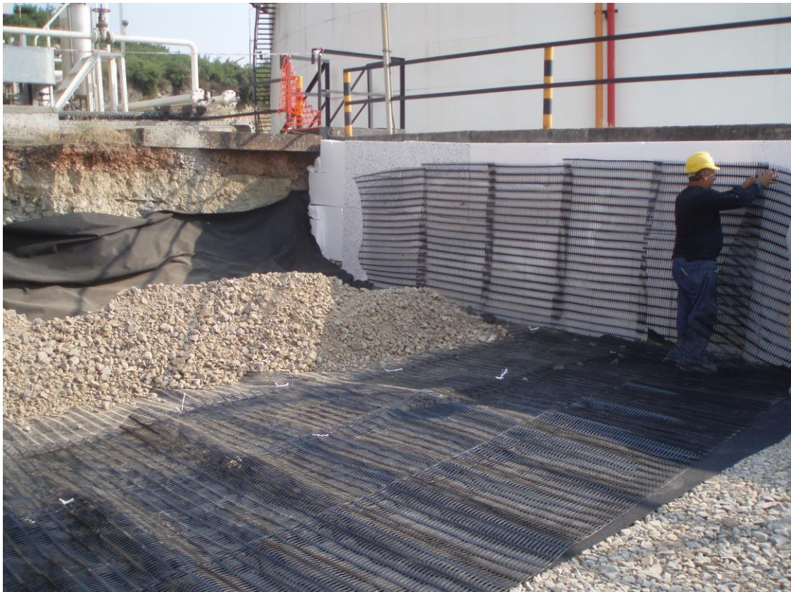
Figure 11: Placement of lowest geogrid layer (and also 1 layer of geotextile)
