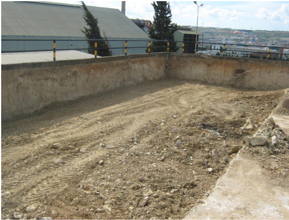
Figure 7: Excavation behind the wall
