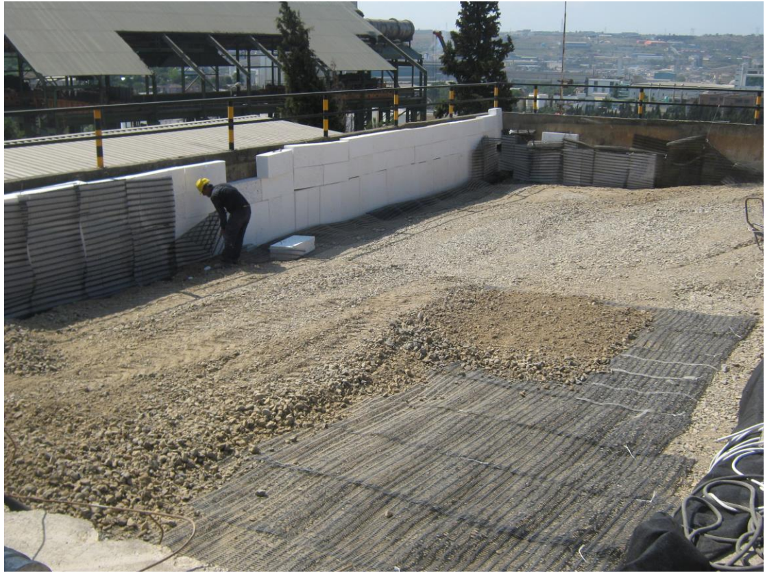
Figure 12: Placement of granular fill over the geogrid
