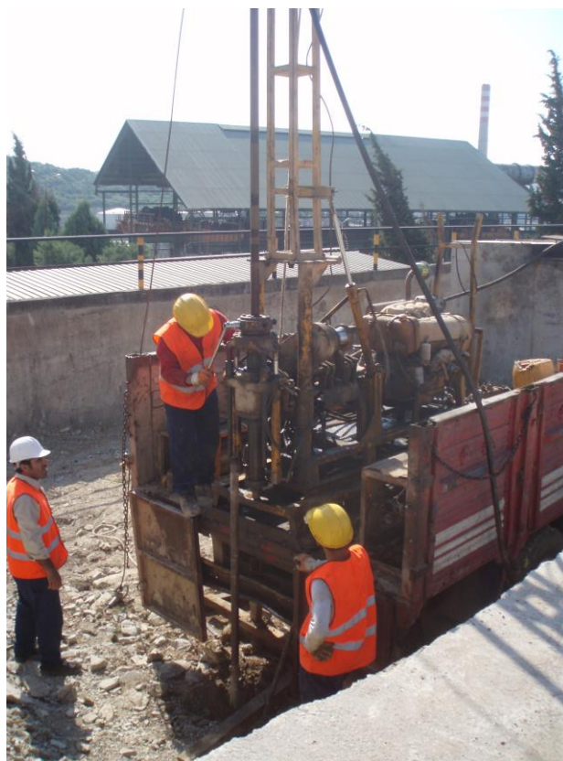
Figure 8: Drilling of boreholes for grouting
