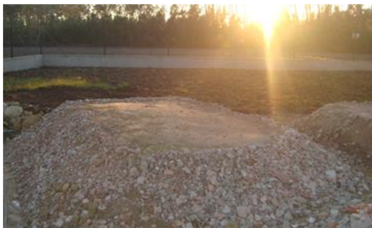
Figure 4: One of the damage trial embankments.
