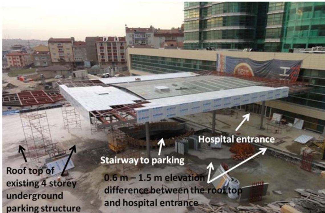
Figure 1: View of the geofoam lightweight fill for flat roof application area
