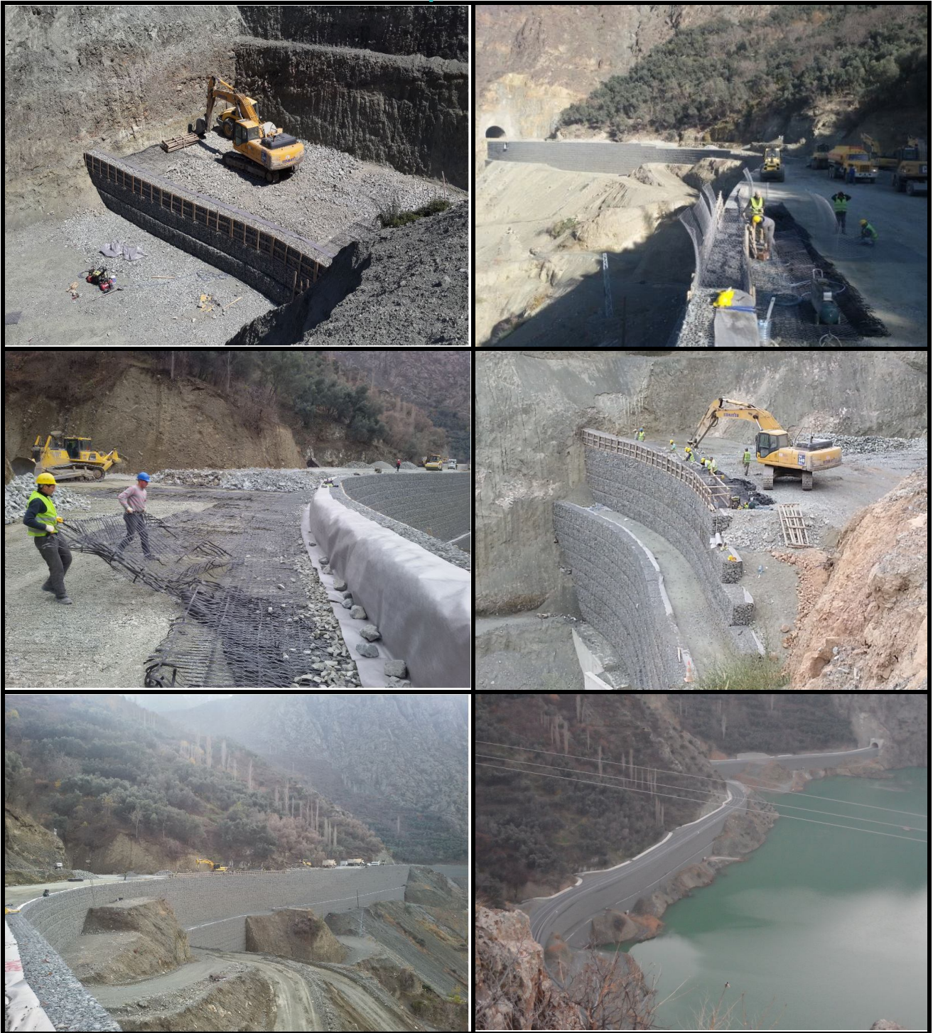
Figure 7. Various stages of the construction and the completed walls
