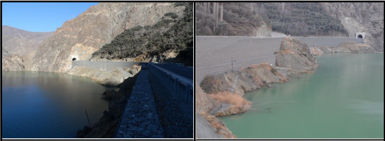
Figure 6. a) Demirkent-2 Tunnel, Demirkent direction
