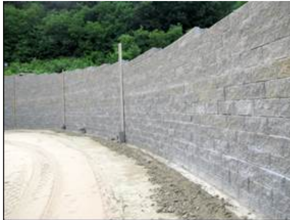
Figure 7. Rebuilt back-to-back reinforced wall with proper materials
