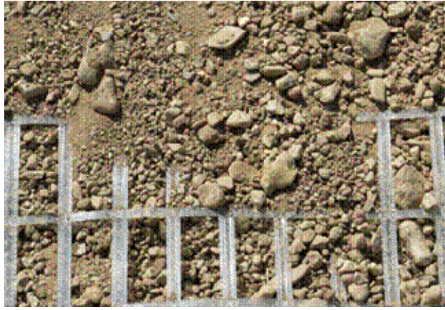
Figure 12. Fill material: more than 88% of the fill material is passing through the openings of the geogrid in absence of a geotextile
