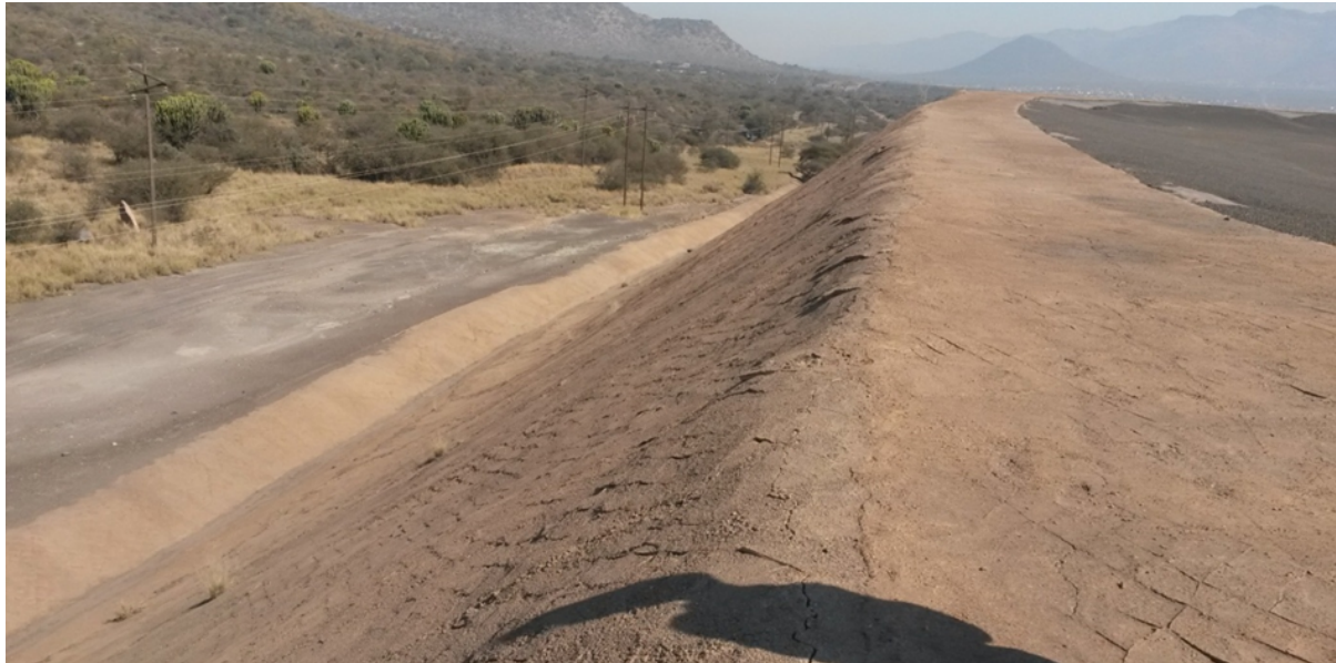
Figure 1. Southern embankment and perimeter drain of existing Capped Facility.
