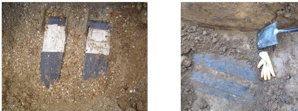
(a) (b) Figure 3: (a) Connection between polymeric reinforcement and concrete facing panel and (b) strap installation
