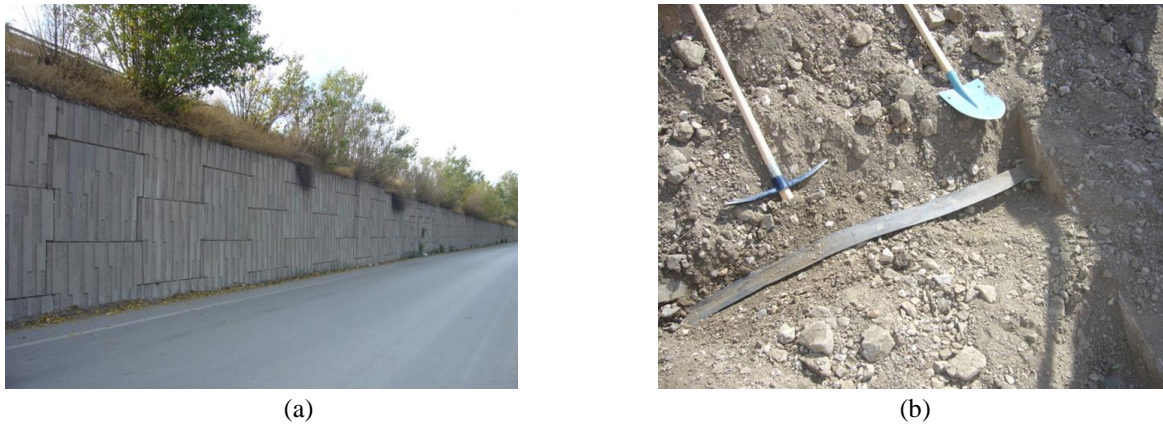
Figure 4: (a) External view of Elmadag wall and (b) exhumation of samples
