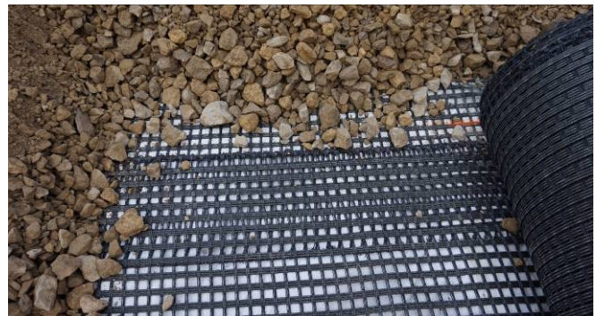
Figure 21 and 22 The reinforcement installation process.
