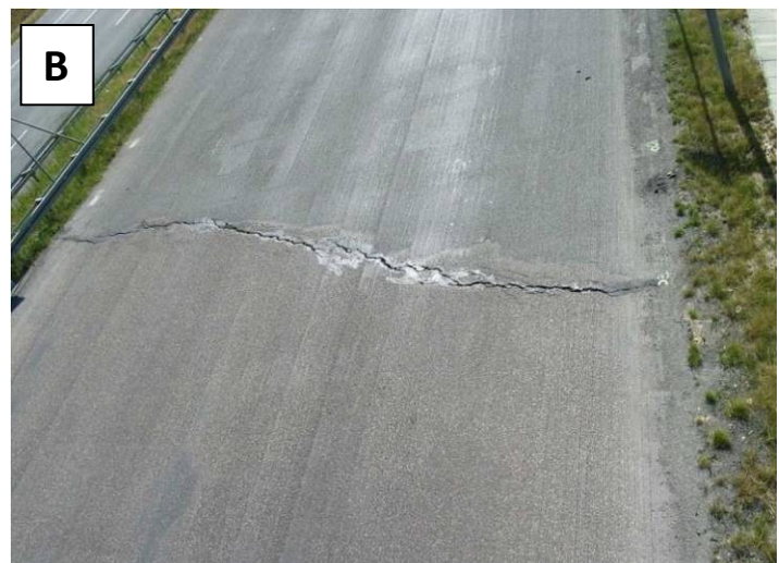
Figure 9. The crack which occurred in 2005.
