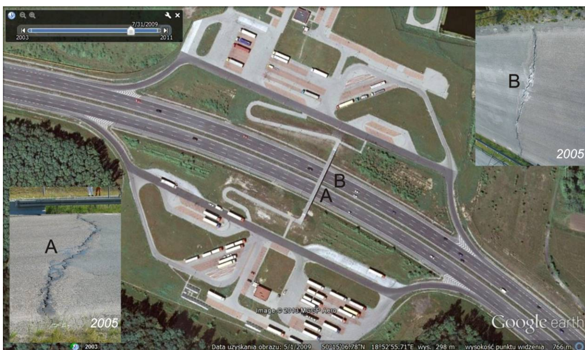
Figure 1. Cracks on the highway surface 2005.
