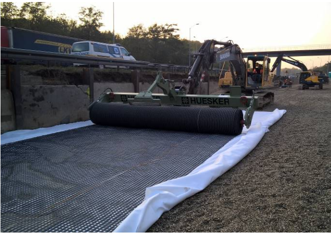
Figure 19 and 20 Geogrid installation process with tension strength measurement.
