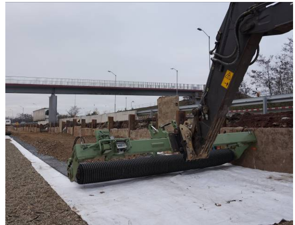
Figure 19 and 20 Geogrid installation process with tension strength measurement.
