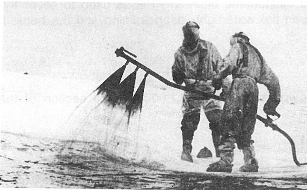
Photo 3. Spraying bitumen by hand
