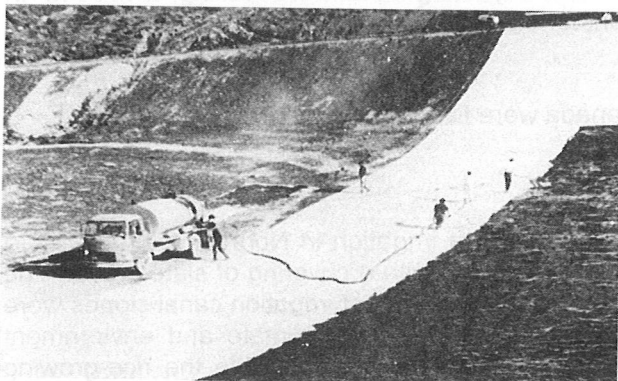
Photo 4. In situ application of bituminous geomembrane reservoir lining
