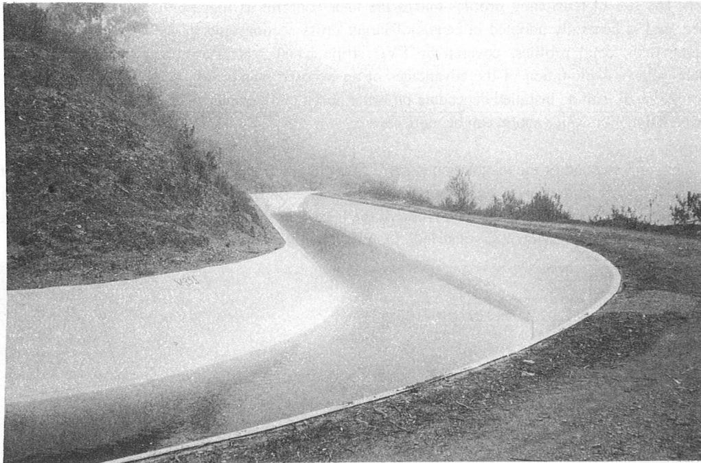
Figure 3. Exposed composite PVC membrane
