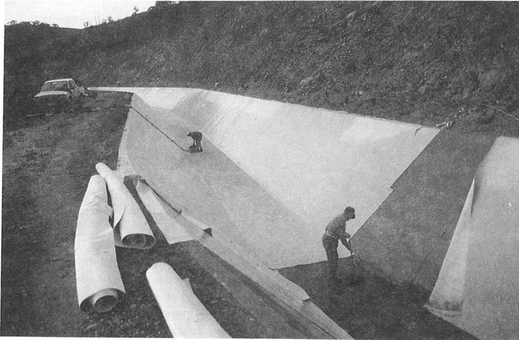
Figure 2. Installation of the PVC waterproofing system at Mira canal
