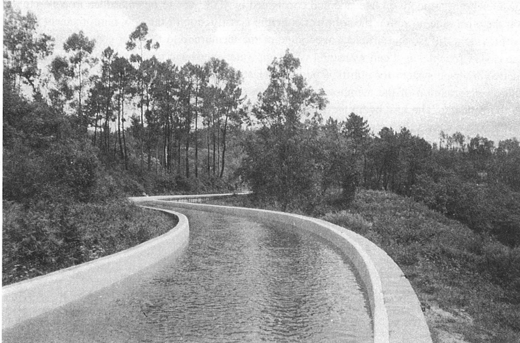
Figure 7. Senhora do Porto canal back in service
