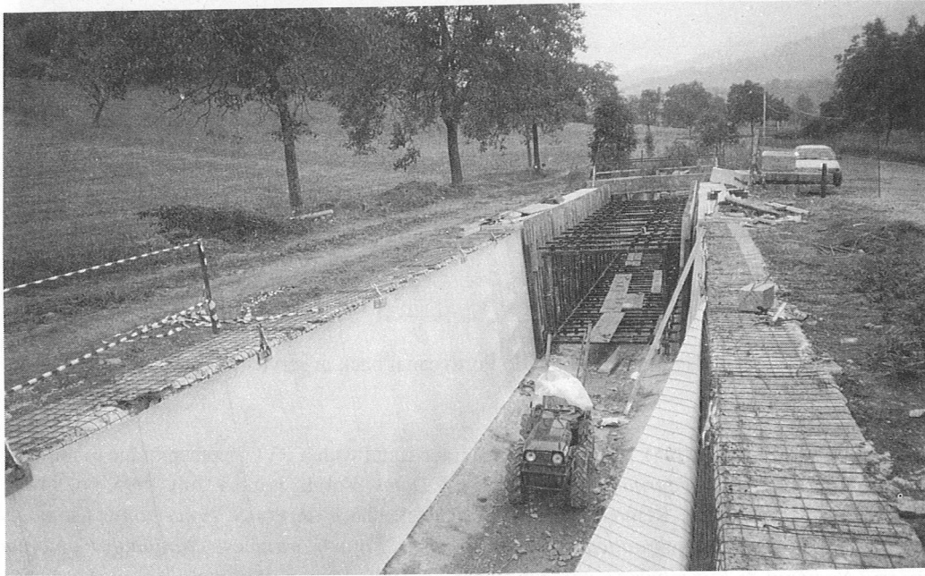
Figure 6. Sibelon CL membrane installed over the Droncro power supply canal
