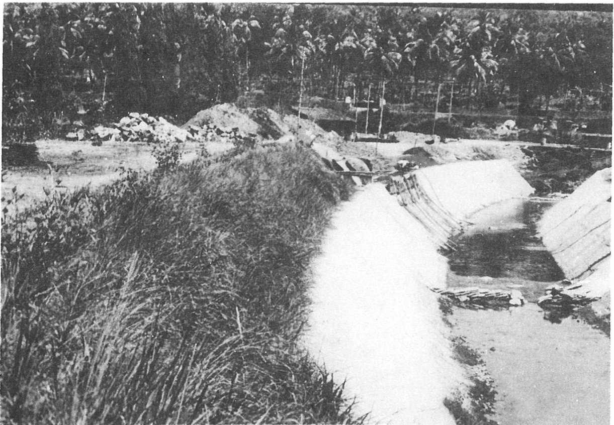
Photo 2: Muvattupuzha (Kerala) Left Bank Main Canal after Geotextile Treatment.
