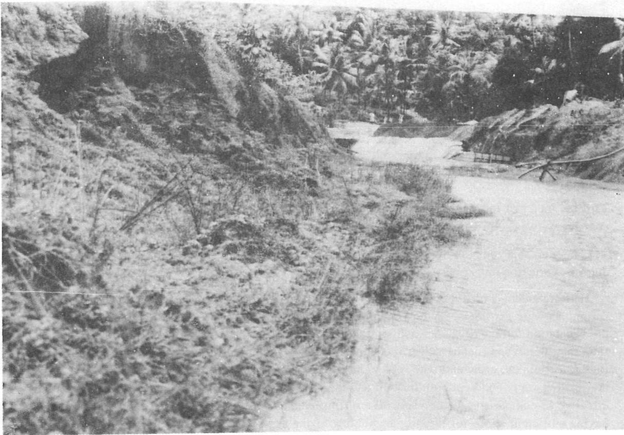
Photo 1: Muvattupuzha (Kerala) Left Bank Main Canal before Geotextile Treatment.
