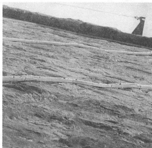
Figure 7. Profiles can also be installed of a very rough substrate, as on masonry dams waterproofed in Italy, France and Switzerland
