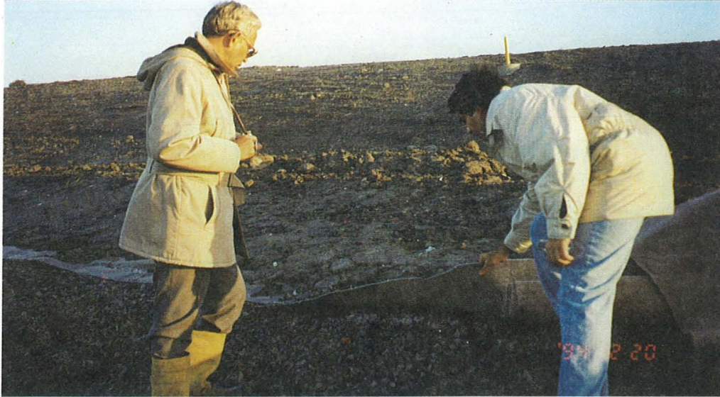
Photo 3 View showing drainage layer overlaid by non-woven geotextile
