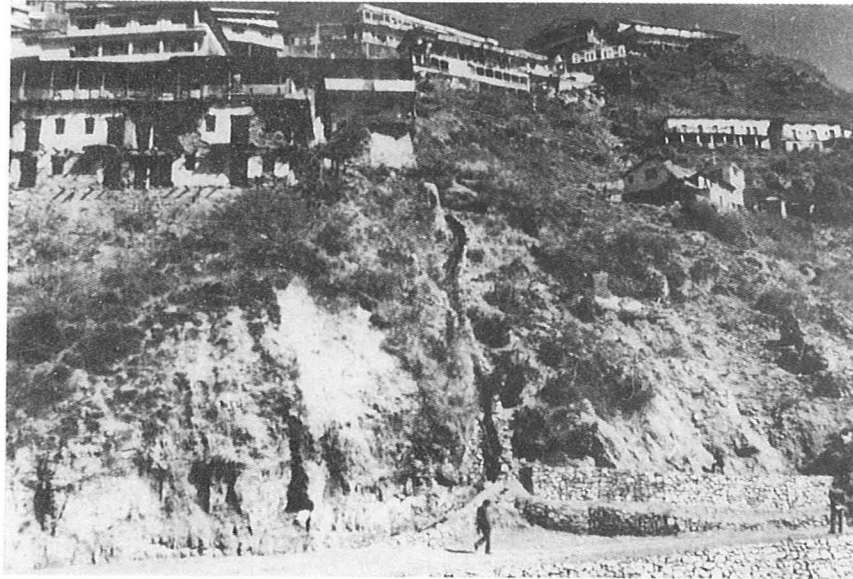
Fig. 2. View of damaged buildings on the slope on Mussoorie-Chamba Bye-pass
