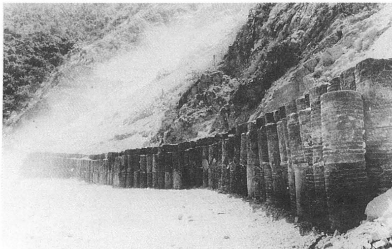
Fig. 8. View of the drum-diaphragm wall built at toe of upper slope
