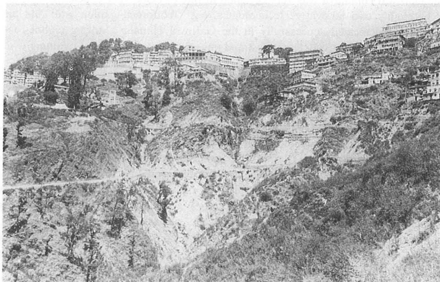
Fig. 1. View of Slope at Km. 5 along Mussoorie Chamba Bye-Pass.
