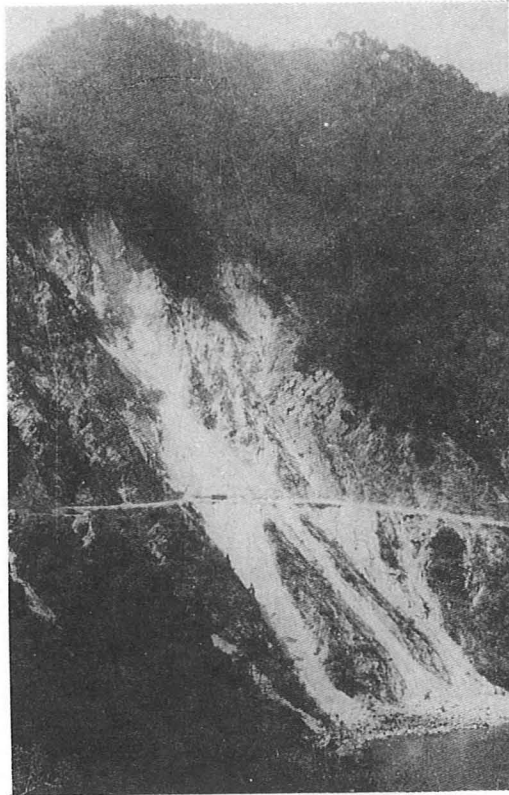
Fig. 5. View of Slope at Kaliasaur landslide
