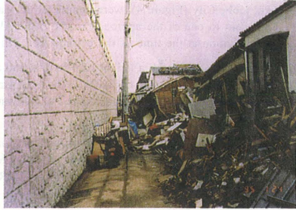
Figure 6: Side view of Tanata wall immediately after the earthquake
