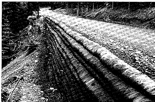
FIGURE 6 Completed Shelton Fabric Wall
