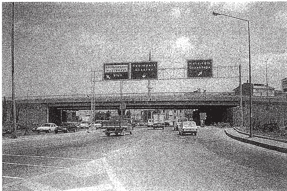
Figure 3. General view of overpass bridge
