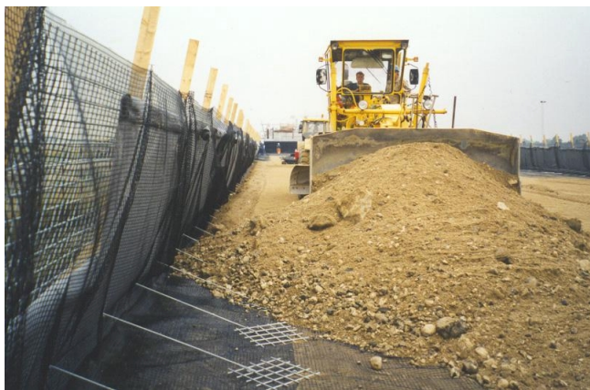
Figure 4. Construction of reinforced fill and facing
