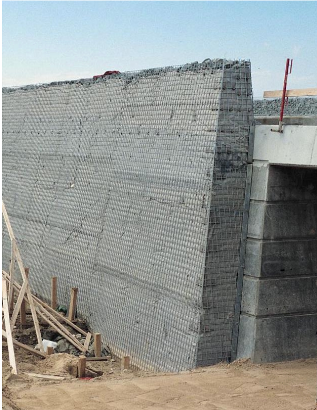
Figure 5 . Green Corner and Parapet in Reinforced Soil
