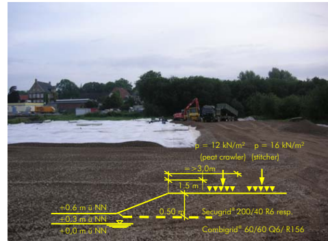
Photograph 6. Installation of the first filling
