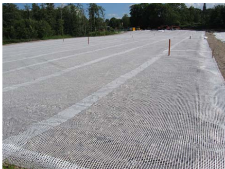
Photograph 8. Installation of the second geogrid layer, Secugrid 60/60 Q1 (polypropylene)
