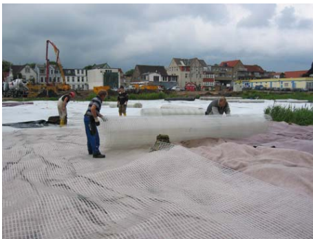
Photograph 5. Installation of Secugrid 200/40 R6 above Secutex R 504
