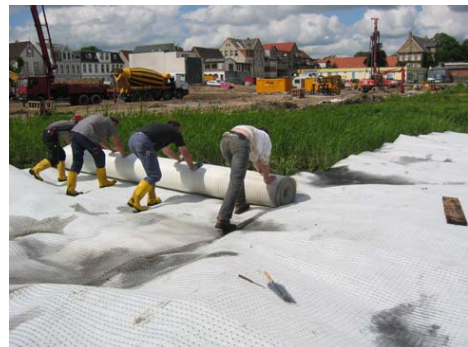
Photograph 4. Installation of Combigrid 60/60 Q6 (polyester) R 156
