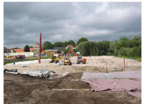
Photograph 7. Installation of the vertical drains
