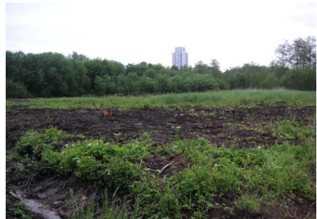
Photograph 1. Construction field after deforestation/clearing works
