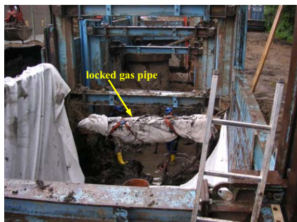
Photograph 3. Soil exchange by means of a guide rail formwork
