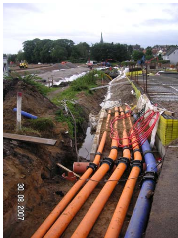
Photograph 2. Re-installation of the service pipes
