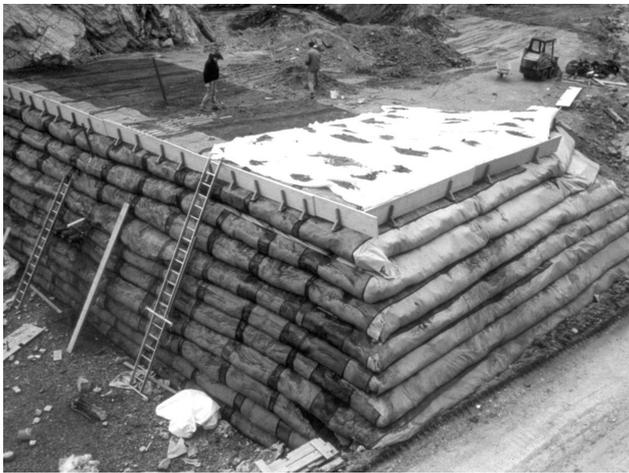
Figures 4 and 5. Construction using steel angles and wooden boards as temporary formwork
