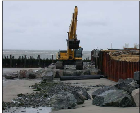
Figure 2. Use of geotextile separation fabric under stone toe fronting a steel sheet pile bulkhead, Strathmere, New Jersey.
