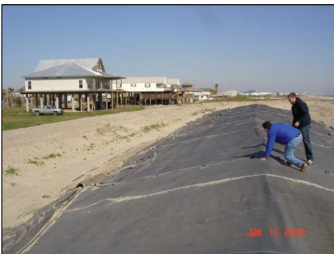
Figure 1. "Geo-burrito" Grand Isle, Louisiana. A woven geotextile was used to wrap a clay core to provide emergency protection.
