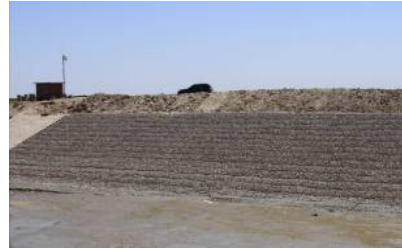
Figure3. Effect after construction with Reno mat
