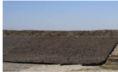
Figure 5 Effects after construction with geocell gravel
