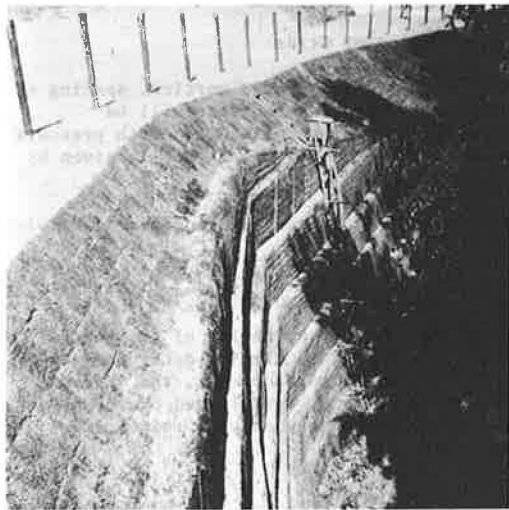
Fig. 8 Completed view of reinforced embankment
