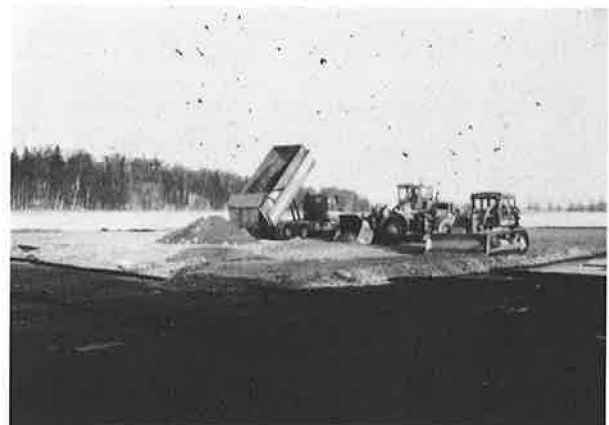
Figure 6 Laying of a protective layer of sand to cover the geotextile
