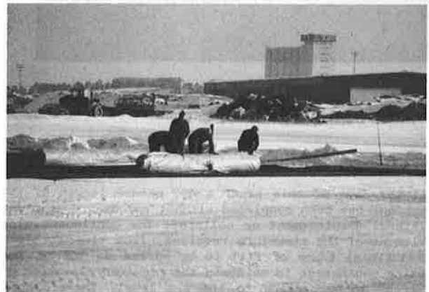
Figure 5 Spreading out of the geotextile on ice
