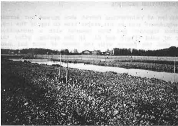
Figure 7 Summer 1984. Ice cap melted. Bordering embankments filled in.
