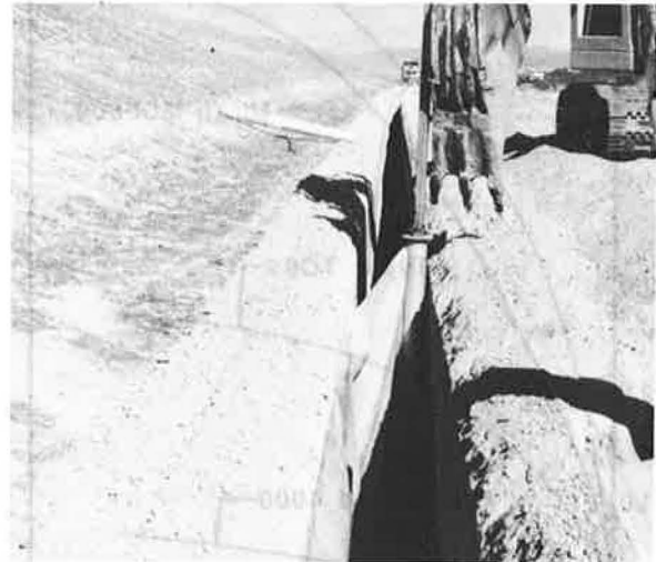
Figure 10: Installation of Downstream Geotextile Cutoff.
